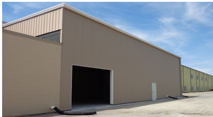
An extension on Distribution Inc.’s building will allow maintenance employees to work on trucks and trailers year-round.
